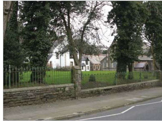
The listed railings around St James's Churchyard
