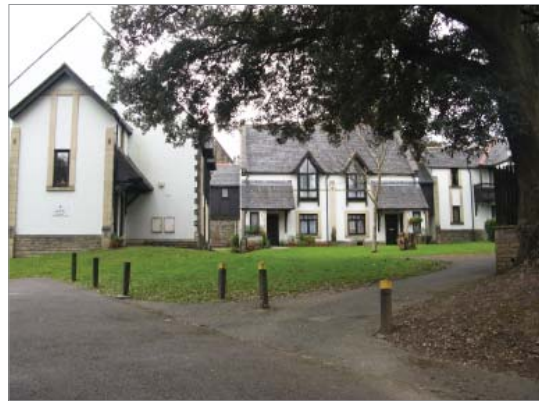
St James' Court, next to St James's Church
